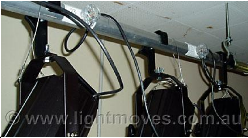
Circuit Tube suspended by Clevis
